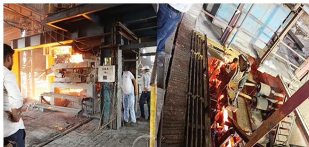
New continuous casting machine (CCM)
